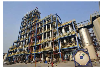
Start up of HFC-125 in Changshu (China)
