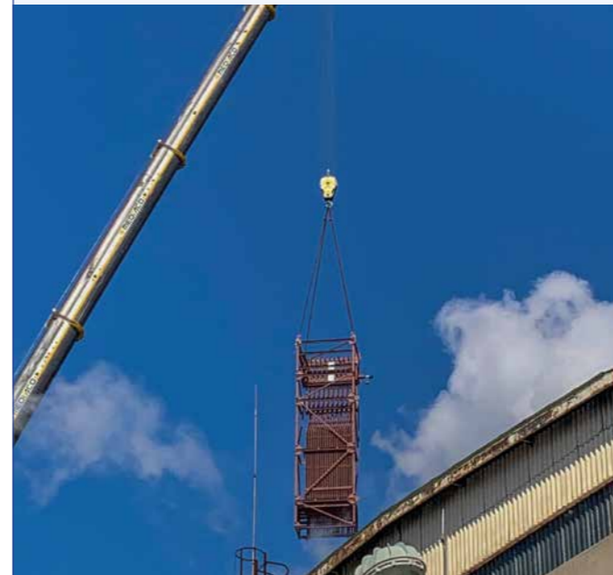
A crane installing the superheater boiler at the Marseille site through the roof of the boiler room
