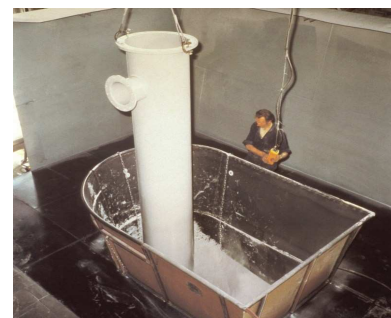
Coating process of pipes in a dipping tank
