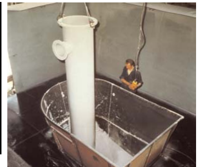
Coating process of pipes in a dipping tank
