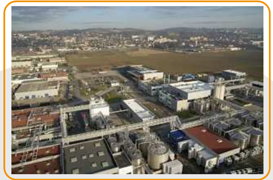
Coatex site in Genay, France
