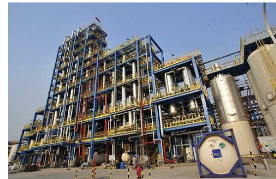
Start up of HFC-125 in Changshu (China)
