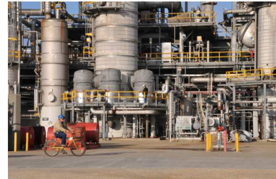
Clear Lake site acquired beginning of 2010 (USA)
